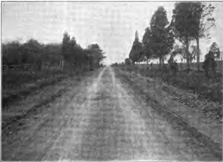
Columbus and Burlington road, Burlington Co., after improvement.
